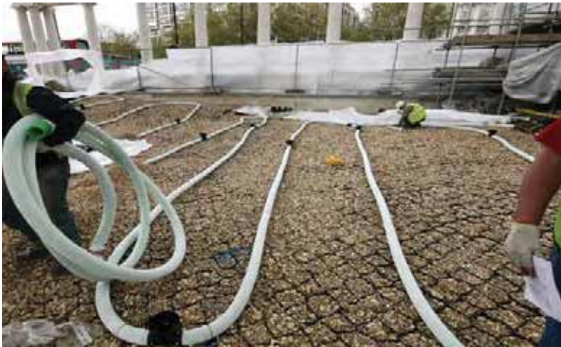
Figure 3. Example of aeration system using perforated piping within the added fill and geoweb layers.
